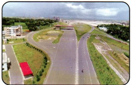
Approach Road and Bridge End Facilities
