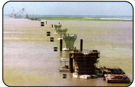
Overall activities of Pier and Pile Cap at Mawa site
