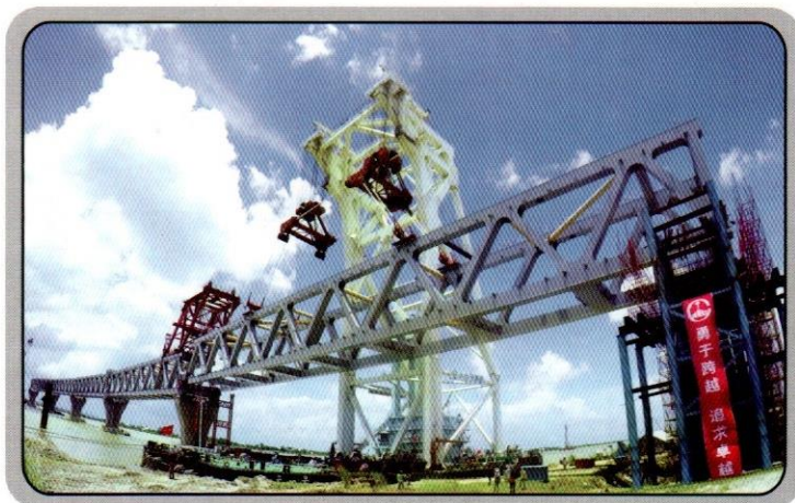
Erection of 5 th Span of the Padma Multipurpose Bridge
