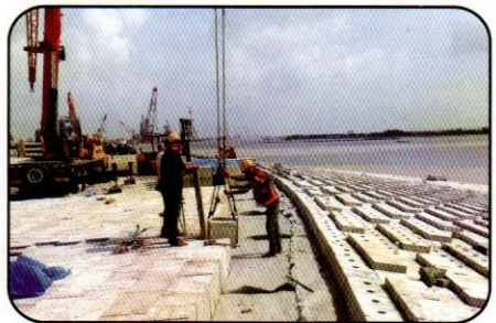
Placement of CC Block at River Site Slope
